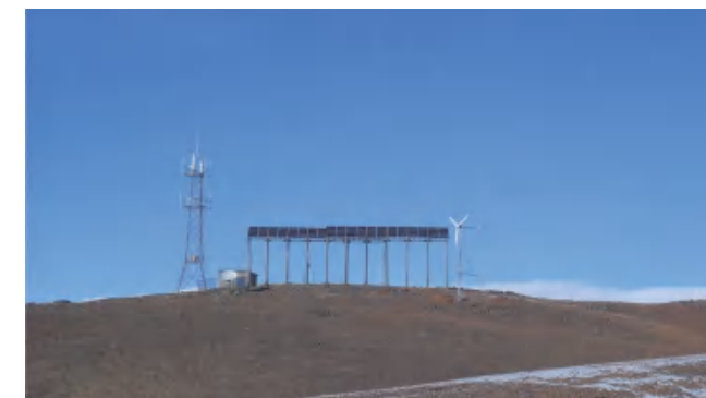
Model: FD5-5 Project location: Heilongjiang Province Run time: 2010 Project description: Solved the power supply problem of base station by wind and PV complementary system
