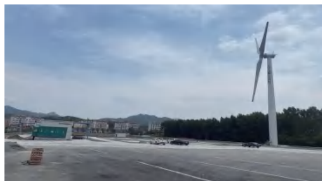
Model: FD56-500kW Project location: Chengde, Hebei Province Run time: 2024 Project description: New energy heavy-duty truck charging station
